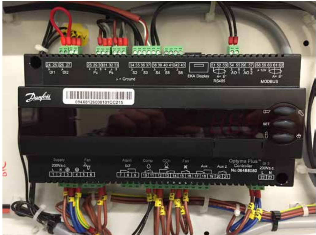
Picture1. Normal wiring
